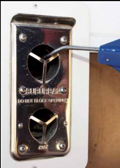
Using an air nozzle, blow air pressure through the intake and exhaust vents from the outside of the coach as part of the annual cleaning.
