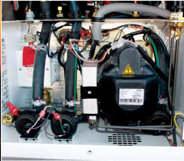
Remove the front cover of the Aqua-Hot once a year and inspect all the components, wires and hoses.
