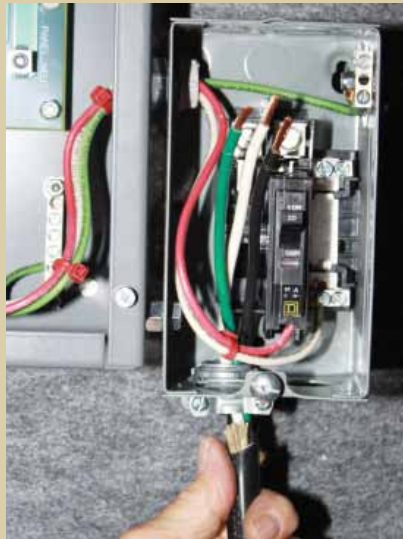
This smaller box houses the 20-amp breaker for the 30-foot power cord. Make sure the cord is securely clamped in place.
