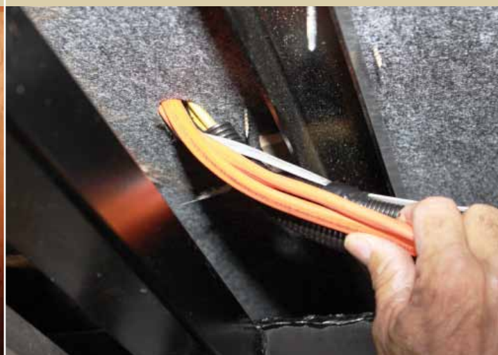
Using an existing access hole located under the floor in the bedroom, we were able to run both Romex wires up to the distribution panel.
