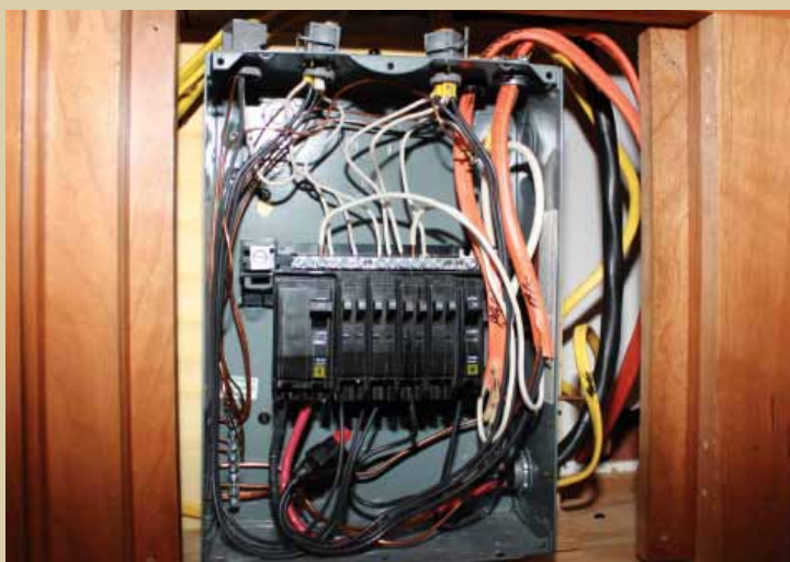
JTB Power Solution labeled both lengths of Romex in the kit, helping take the guesswork out of the connection process inside the main distribution panel of the coach.
