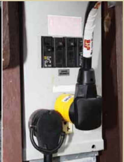
The JTB power cord with adapter is plugged into the GFCI, alongside the 30-amp power cord from the RV.
