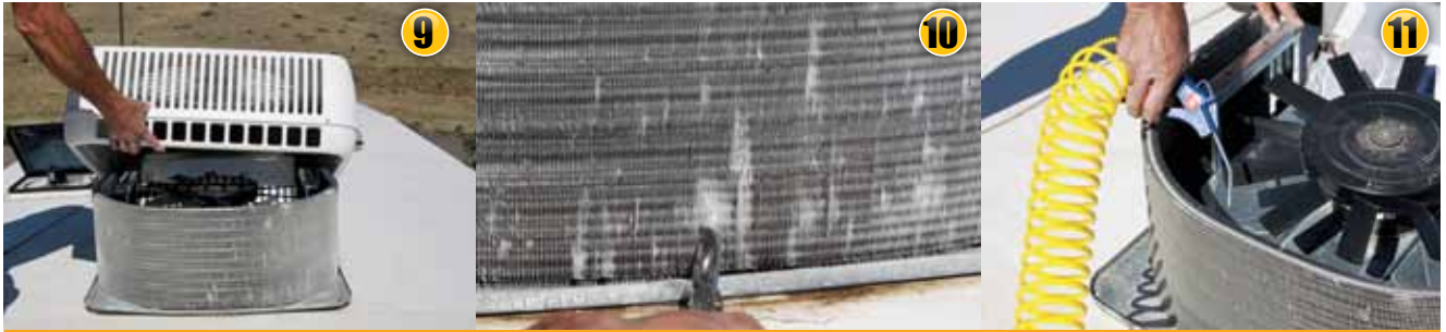
9) Annual A/C maintenance includes removing the shroud and inspecting condenser and wiring. 10) Check condenser for debris or bent fins. For optimum performance, straighten damaged fins using a thin tool. Use an evaporator comb if damage is extensive. 11) Clean condenser with low air pressure, taking care not to damage the delicate fins. A clean condenser makes the A/C more efficient.
